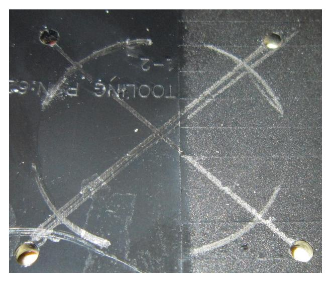
Measure the distance between the center of the fan to the opening.
