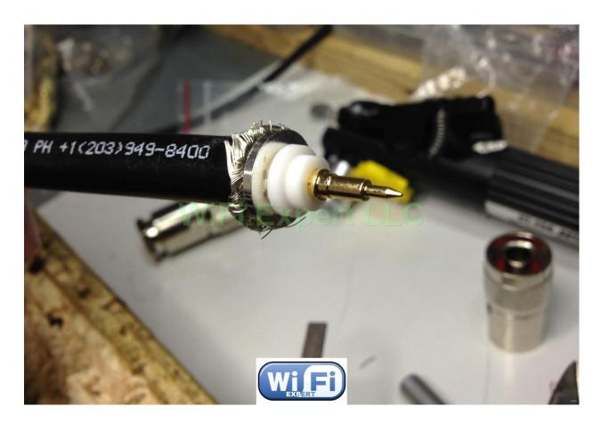
STEP 6: INSTALL THE REST OF THE CONNECTOR.
