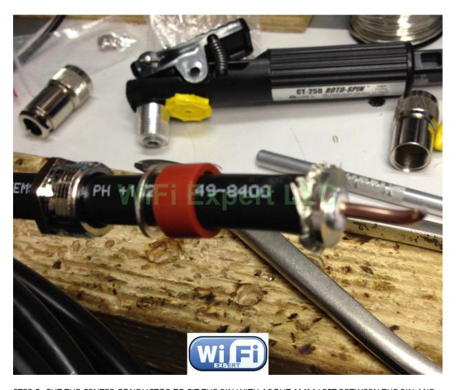
STEP 5: CUT THE CENTER CONDUCTOR TO FIT THE PIN WITH ABOUT 1MM LEFT BETWEEN THE PIN AND THE ISSOLATION PART OF THE CABLE. PLEASE NOTE SOME CONNECTORS MIGHT NEED TO BE SOLDERED AND SOME ARE EZ TYPE (SLIDE ON ONLY). REMOVE THE PIN FROM THE PLASTIC CASING IF REQUIRED TO SOLDER.
