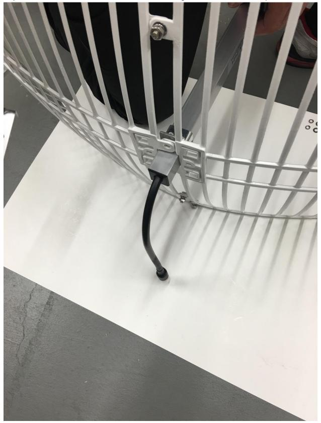
Step 3: Insert the feed into the middle location and use Longer screws to secure it in to place.
